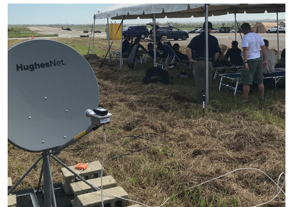
Hughesnet provides connectivity to the airfield at the San Juan Airport.
