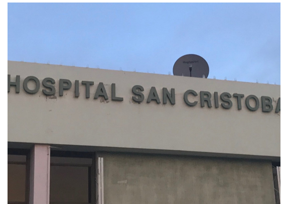
A Hughes VSAT solution installed on the roof of the Hospital San Cristobal made connectivity possible.
