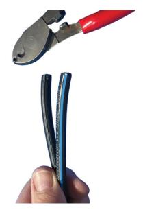
Figure 55: Splitting the IFL cable to length
