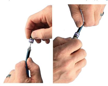
Figure 61: Inserting the IFL cable into the connector
