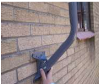
Figure 28: Pole assembly
