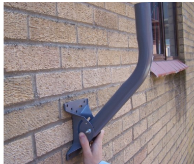
Figure 29: Pole assembly
