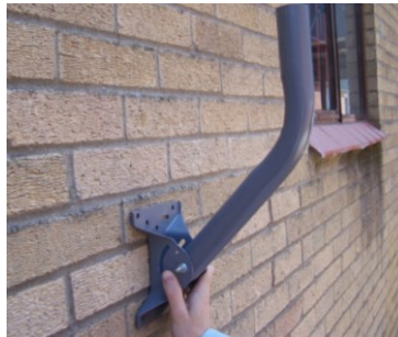
Figure 30: Pole assembly
