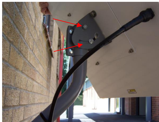
Figure 42: Adjusting elevation
